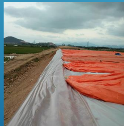
边坡隔水膜铺设
